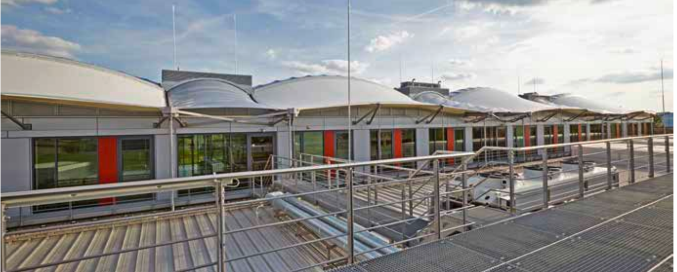
Das Energy Efficiency Center in Würzburg
