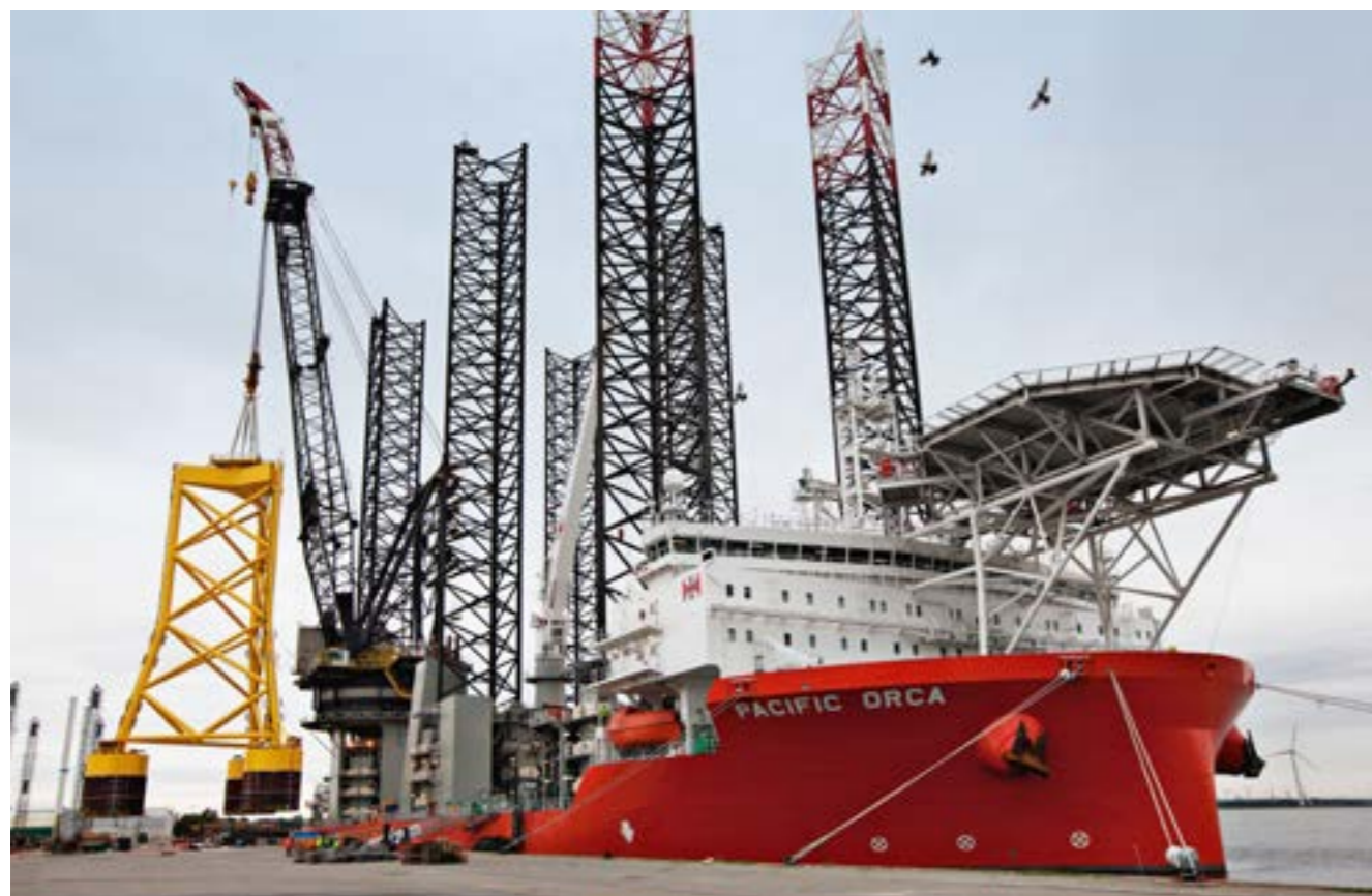
Suction-Bucket-Fundament von Dong Energy.
