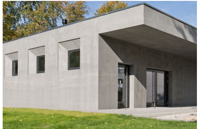
Betonoase – construction project made of infralight concrete
