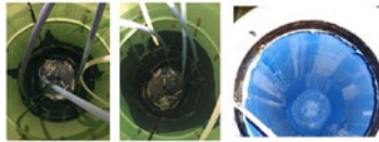
4. waterproofing and curing
