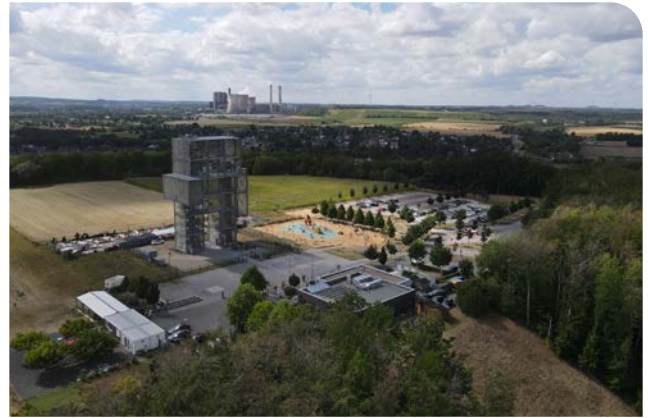
New innovative hydrogen technologies are being developed in the Helmholtz Cluster.
