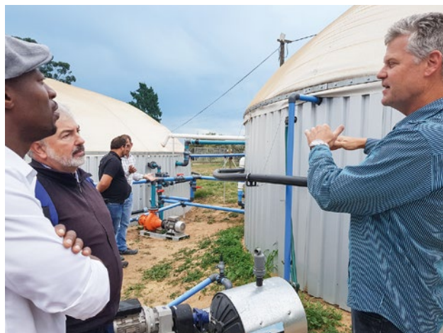
Tour of a biogas plant in Paarl, South Africa
