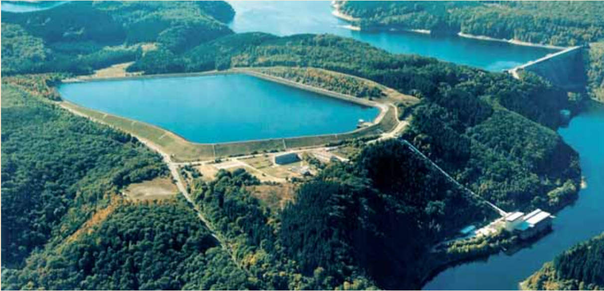
Wendefurth pump-fed power station.
