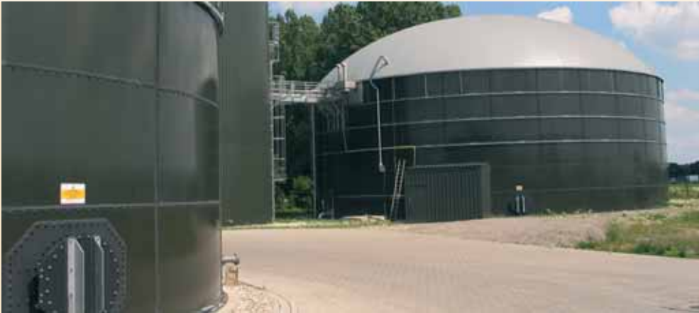
Biogas plants, important balancing elements in load management.
