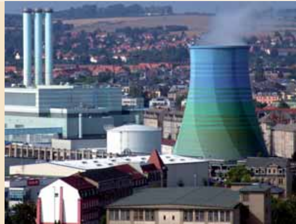
Modern DREWAG CHP plant.
