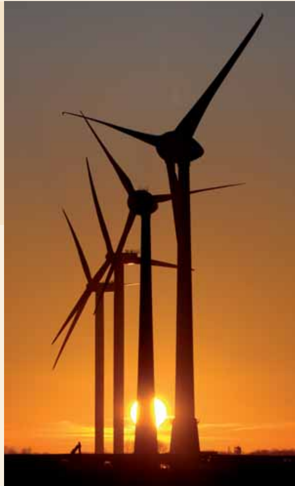
Wind power plants in the offshore test field in Cuxhaven. The “wind harvest” is to be on offer on the eTelligence marketplace in the future.
