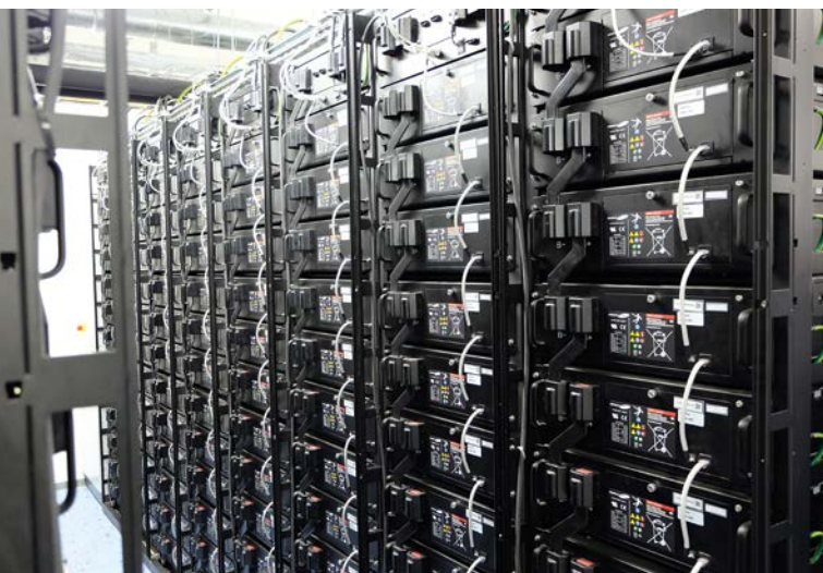
Figure 20: Lithium-ion storage batteries in standardised industrial racks
