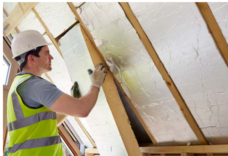
Figure 27: Installing interior insulation
