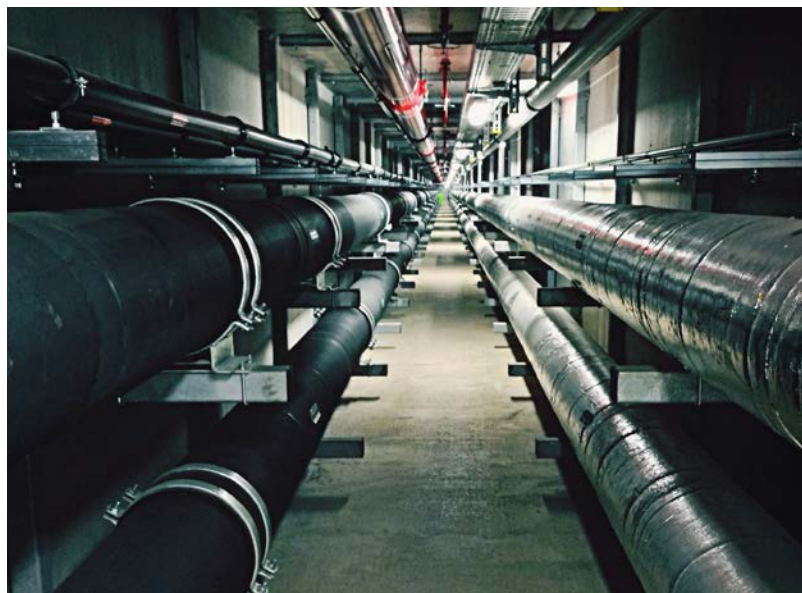
Figure 24: District heating tunnel
