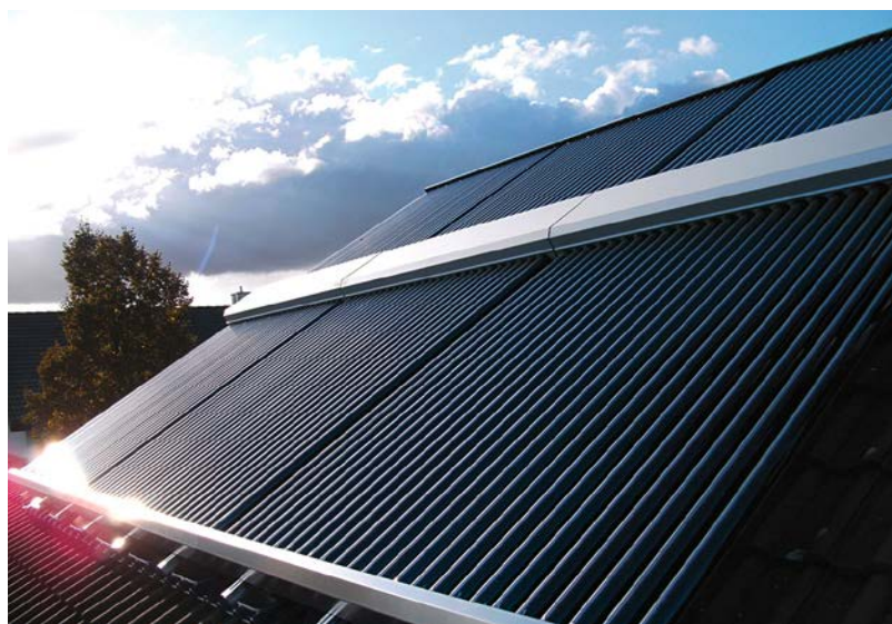
Figure 13: Solar heating collector
