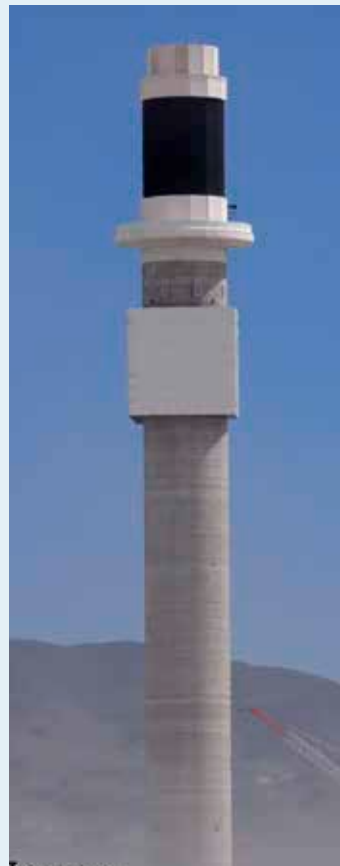
Receiver at the salt tower power plant “Crescent Dunes” in the USA
