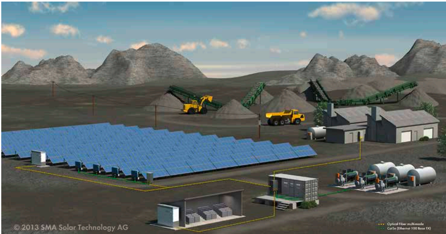
PV/diesel systems with PV, battery storage and diesel generators for the independent supply of a small off-grid facility (in this case a mine)
