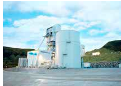
Recycle-to-Gas plant from the project ecoloop® (see page 107)
