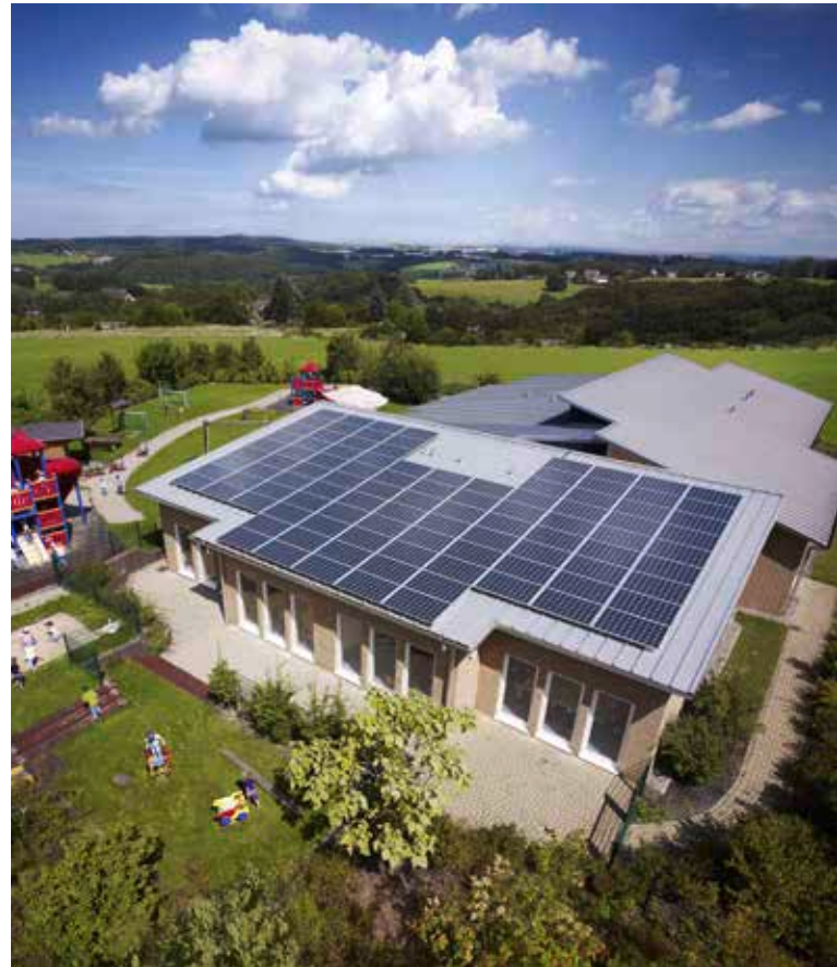
100 SolarWorld PV modules on the roof of the day-care centre Kalenborn in Rhineland-Palatinate save 9.7 tonnes of greenhouse gases per year and generate 17.6 megawatt hours of electricity.
