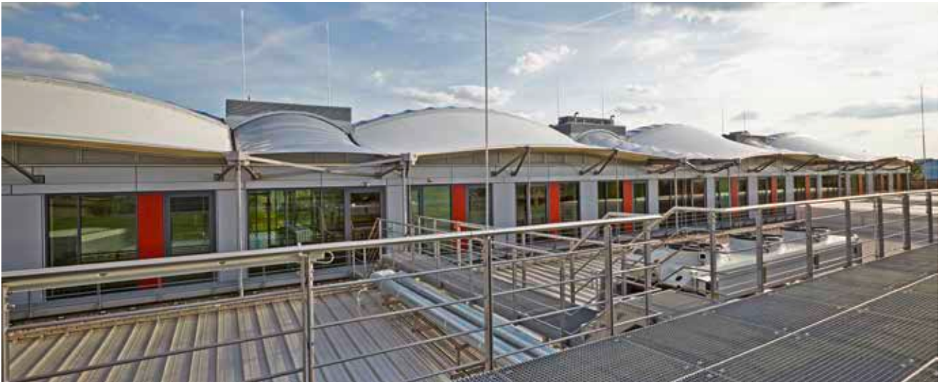
The Energy Efficiency Center in Würzburg
