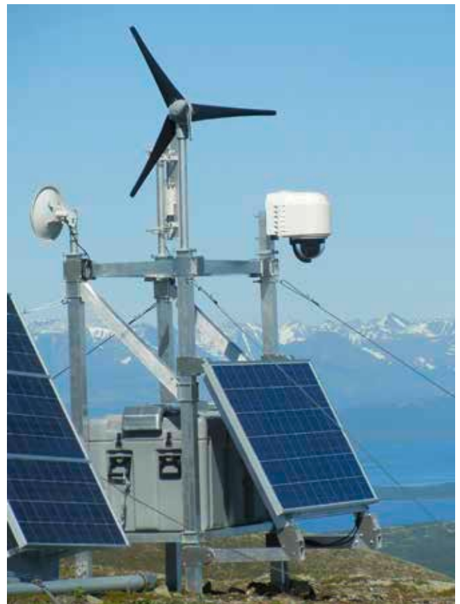
Application of the EFOY ProEnergyBox, a complete off-grid energy solution with an integrated EFOY Pro fuel cell, fuel cartridges and batteries
